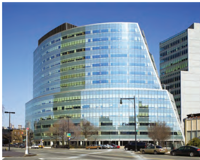
Two Court Square, Long Island City, NY, designed by Kohn Pedersen Fox
